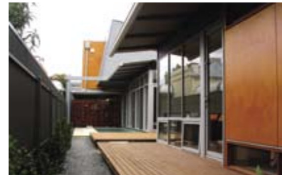
Foundry House Swanbury Penglase
